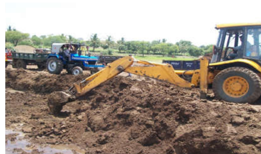
Desiltation in progress
